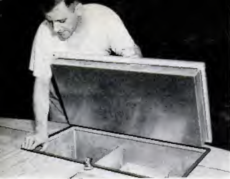
Weather stripping provides a seal for ice-box cover
